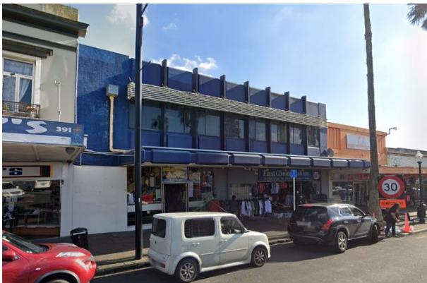
Figure 9: 387 Great South Road (Google Street View, August 2020)
