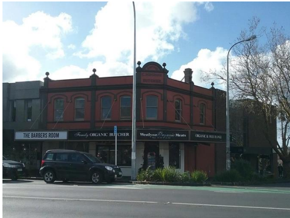
Figure 1: C. Norgrove Butcher building, 428-440 (438-440) Richmond Road
