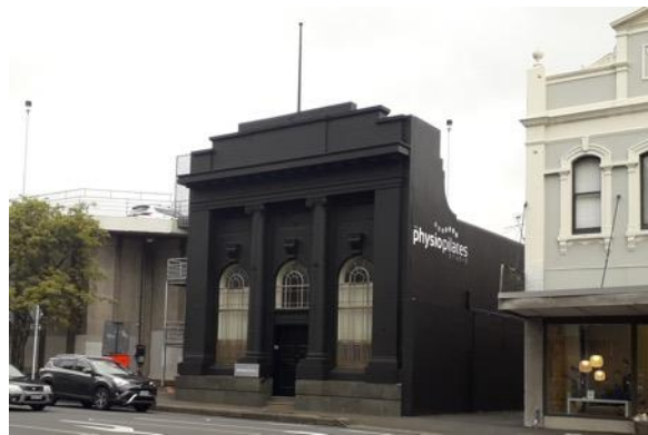
Figure 4: Former ASB Bank, 29 Khyber Pass Road
