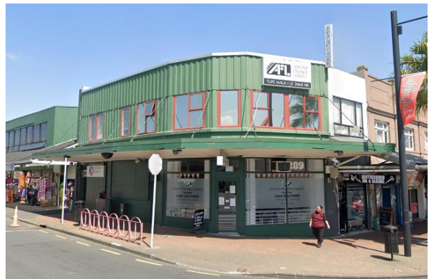
Figure 10: 289 Great South Road (Google Street View, August 2020)
